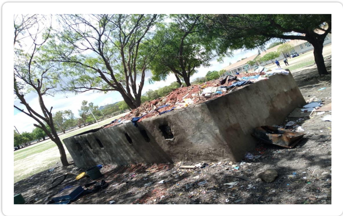
Figure 4. 10: School B's Waste-Disposal Pit
